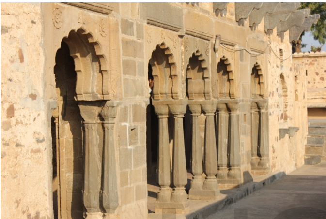
FIG 6. CERTAIN BUILDING ELEMENTS RESTORED FROM OLD DILAPIDATED HAVELIS AND REUSED IN A NEW FORM.
